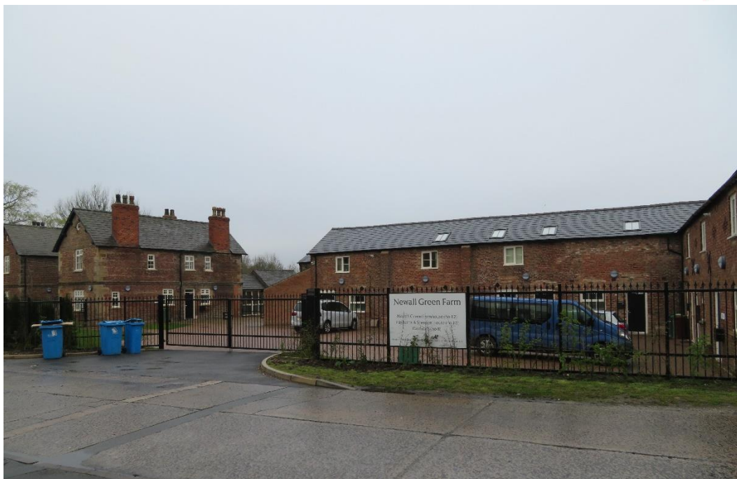
Plate 2: Former threshing barn, with the later stables to the right
