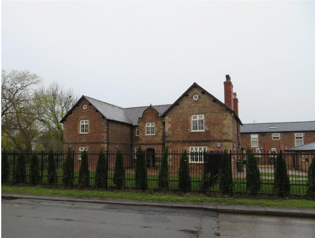
Plate 1: Newall Green Farmhouse, with the former shippon to the rear and right
