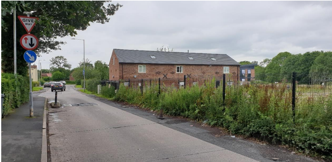
Plate 4 The north-eastern elevation of the stables. The views of these historic buildings can be appreciated from Barnacre Avenue due to the lack of development on the western side of the road
